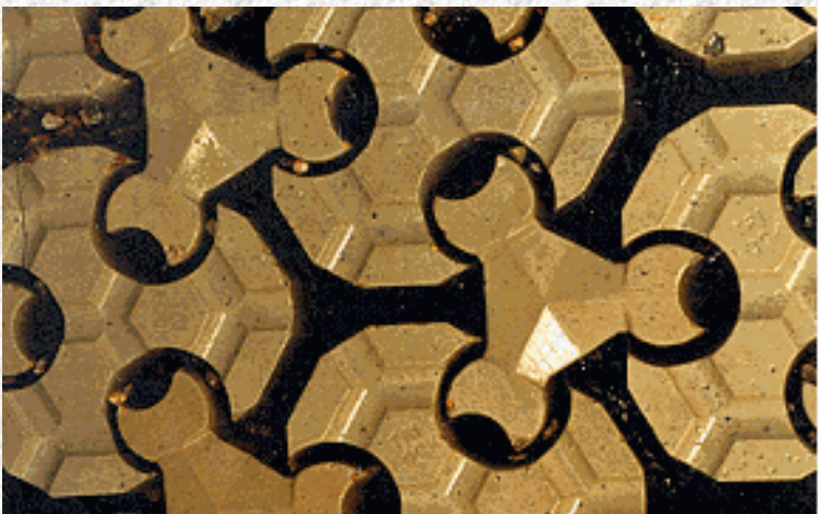
Figure 4.1 Examples of Interlocking Block and Cable-Tied Block Systems (left, courtesy American Excelsior; right, courtesy Armortec)
