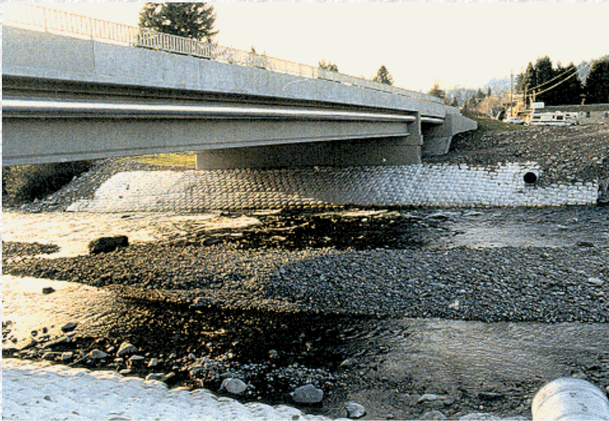
Figure 5.5 ABM Installed on West Bank of Salmon Creek (ODOT)
