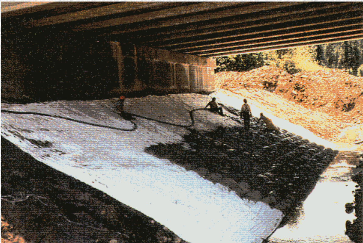
Figure 5.3 Installation of Articulating Block Mat Proceeding Upslope (ODOT)
