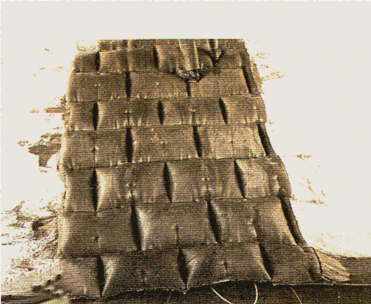
Figure 5.1 Articulating Block Mat Appearance after Filling (ODOT)
