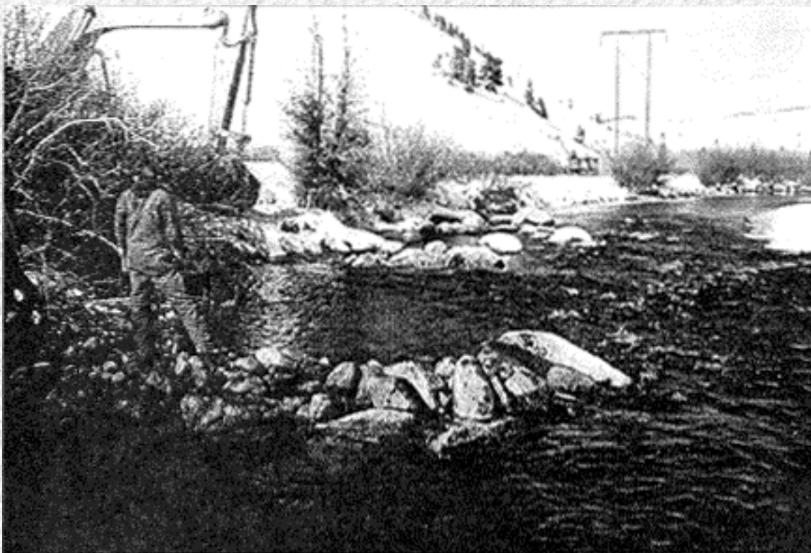
Figure 1.4 Bendway Weirs Installed on the Blue River Near Silverthorne, Colorado (CDOT)
