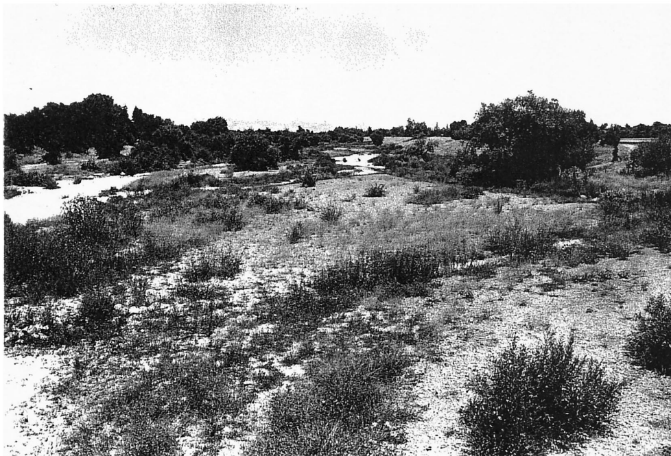
Figure 5. Photographs looking downstream from Santa Teresa Bridge at the channel of Uvas Creek. (a) in January 1996, about 2 months after construction of the channel reconstruction project, and (b) in June 1997, after the project had washed out. (1996 photograph courtesy of the City of Gilroy, 1997 photograph by Kondolf.)
