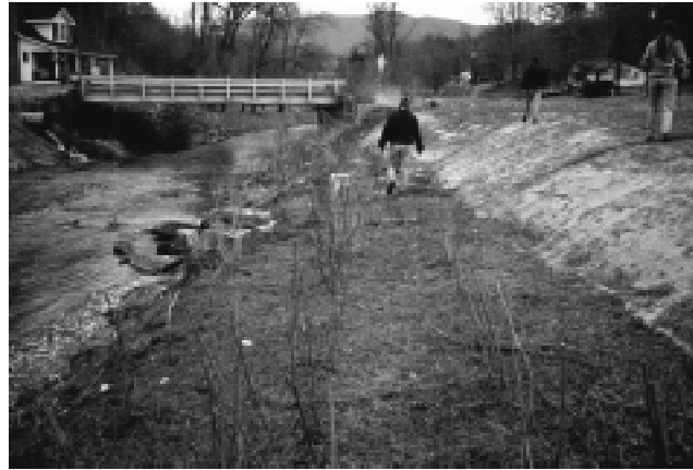
Figure 1. Many streams in the North Carolina mountains and piedmont are incised. The potential for erosion increases as streambank height increases. These incised and eroding streambanks should be graded to include a bankfull bench.
