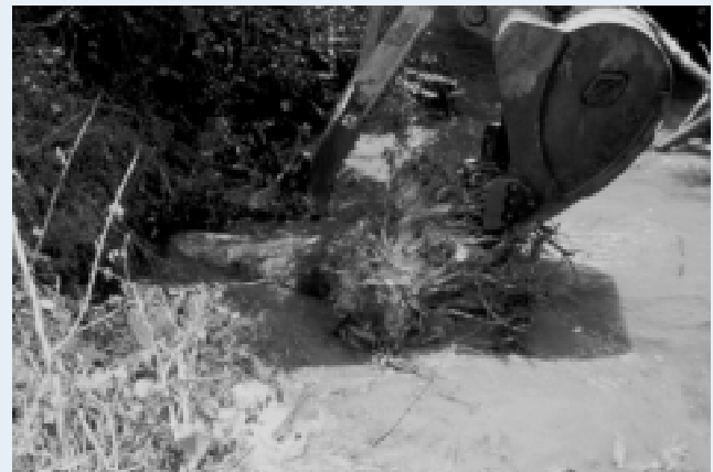
Figure 3. Root wad installation using drive-point method.
