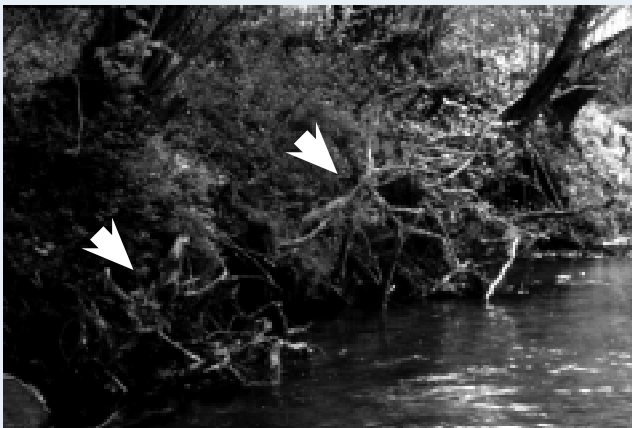
Figure 2. Root wads after installation.
