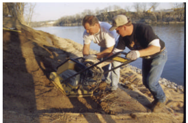
Figure 1. Soil is compacted after installing a brushlayer lift. Correct compaction is needed after material installation to close voids and to provide suitable soil density for appropriate plant growth
