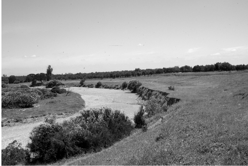
Figure 4. Buckeye Creek, before Bendway Weirs.
