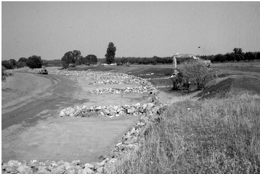
Figure 5. Bendway Weirs, during completion of the keyways landward of the LPSTP.
