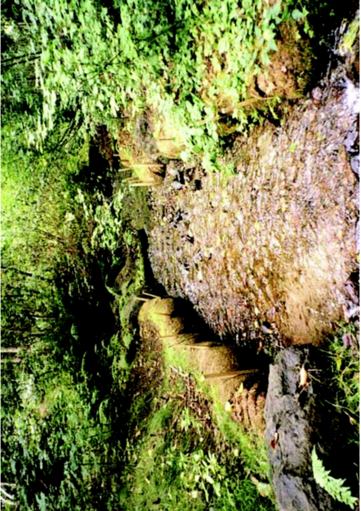
Figure 6-37. Coir Logs. Zaccuse Creek, Tributary to Lake Sammamish. 2000. Source: King County Department of Natural Resources.
