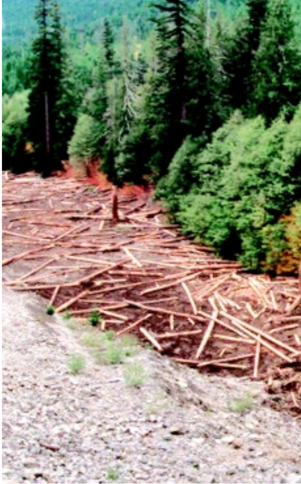
a. Floodplain Roughness using large woody debris. Clearbranch Creek, OR. Source: Inter-Fluve, Inc.
