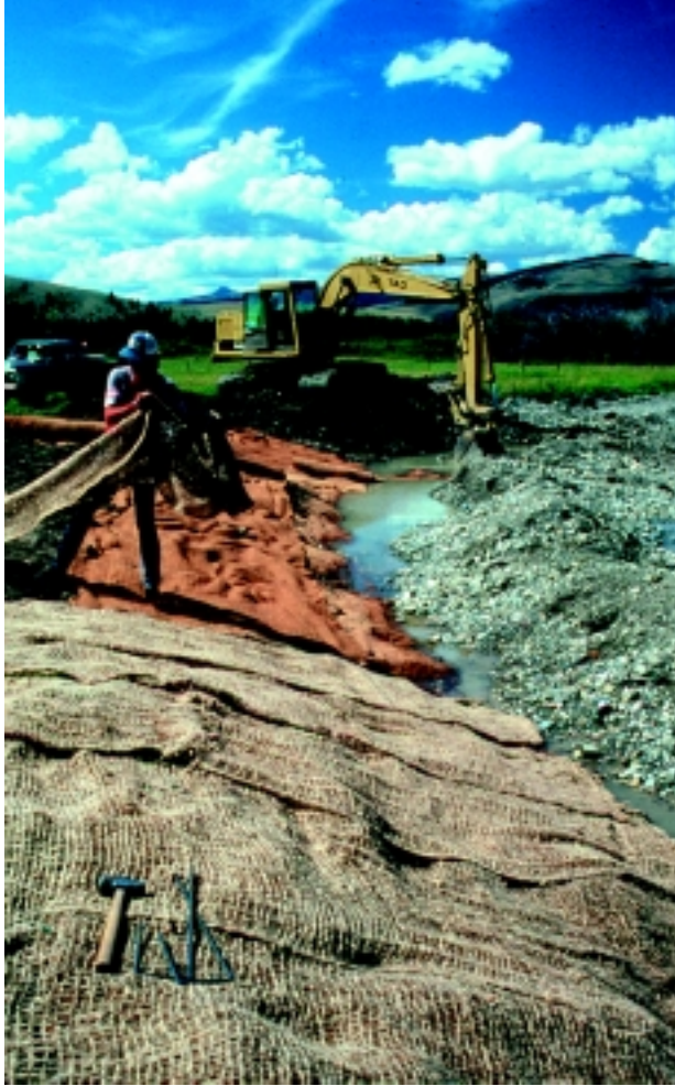
a. Bank reshaping. Unidentified creek in Montana. Source: Inter-Fluve, Inc.
