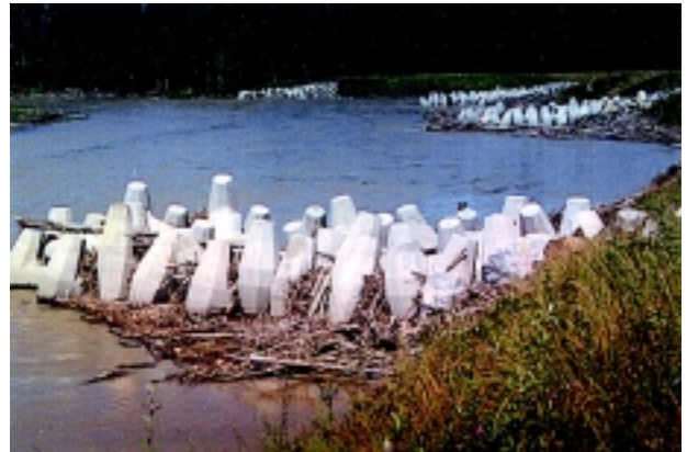
e. Dolo Groins. Nooksack River. 1998. Source: Inter-Fluve, Inc.
