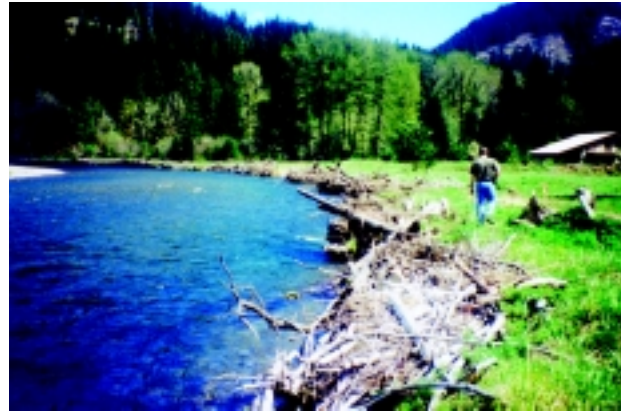
d. Wood Groins. Wind River. One year after construction. Note wood accumulation. 2000.
