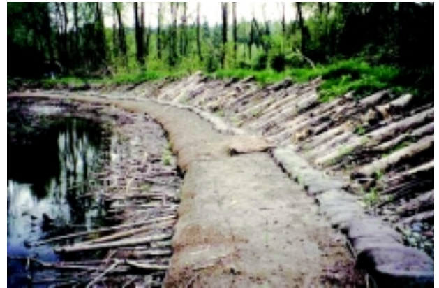
d. Soil Reinforcement lifts with woody plantings. Cedar River side channel.
