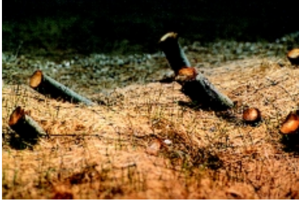
a. Live Stakes planted through Coir Fabric. Source: Inter-Fluve, Inc.
