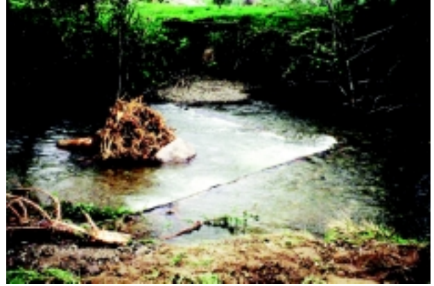
c. Vee Log Drop Structure. Little Hoko River, Tributary to Strait of Juan De Fuca. 1996.
