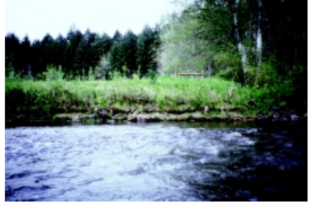
d. Roughened-Rock Toe with reinforced soil lifts and plantings. Deschutes River. 1996.
