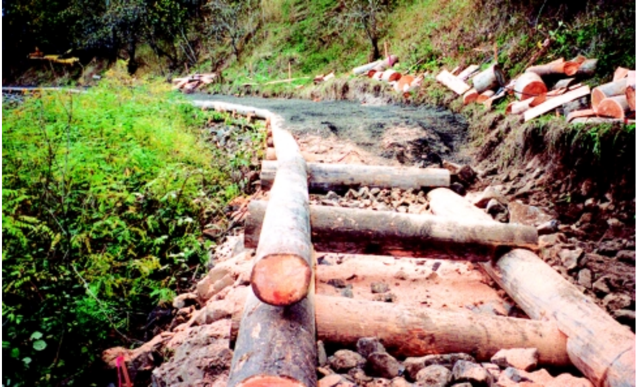
a. Log Cribwall during construction. Columbia River. Source: Inter-Fluve, Inc.
