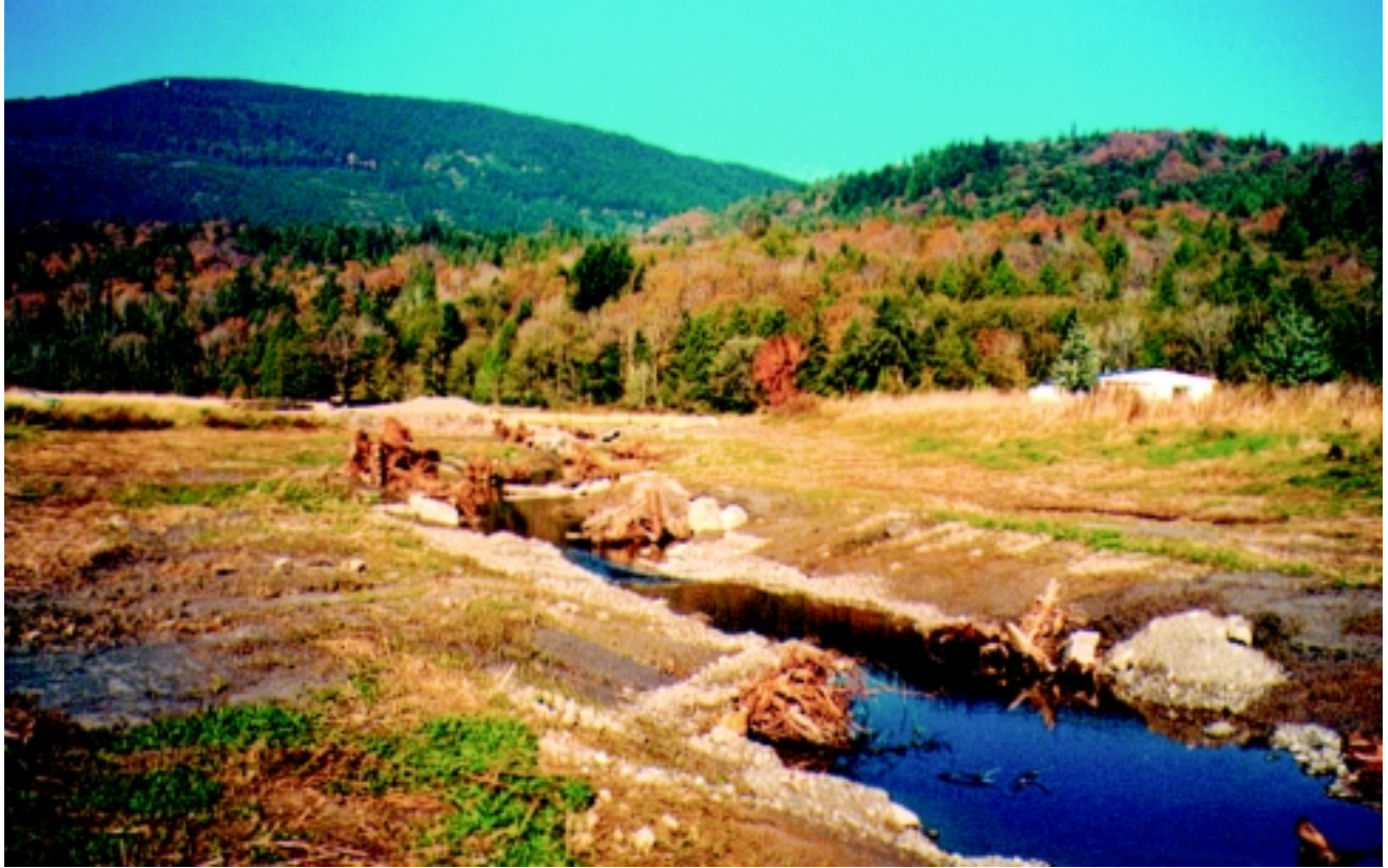
a. Channel Relocation to restore a channelized and eroding stream. Colony Creek, Tributary to Samish Bay, Puget Sound. 1999.
