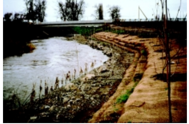
c. Soil Reinforcement lifts with rock toe. Touchet River. 2000.
