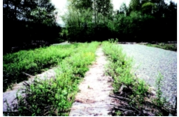
c. Rows of Woody Plantings. Cedar River Levee.
